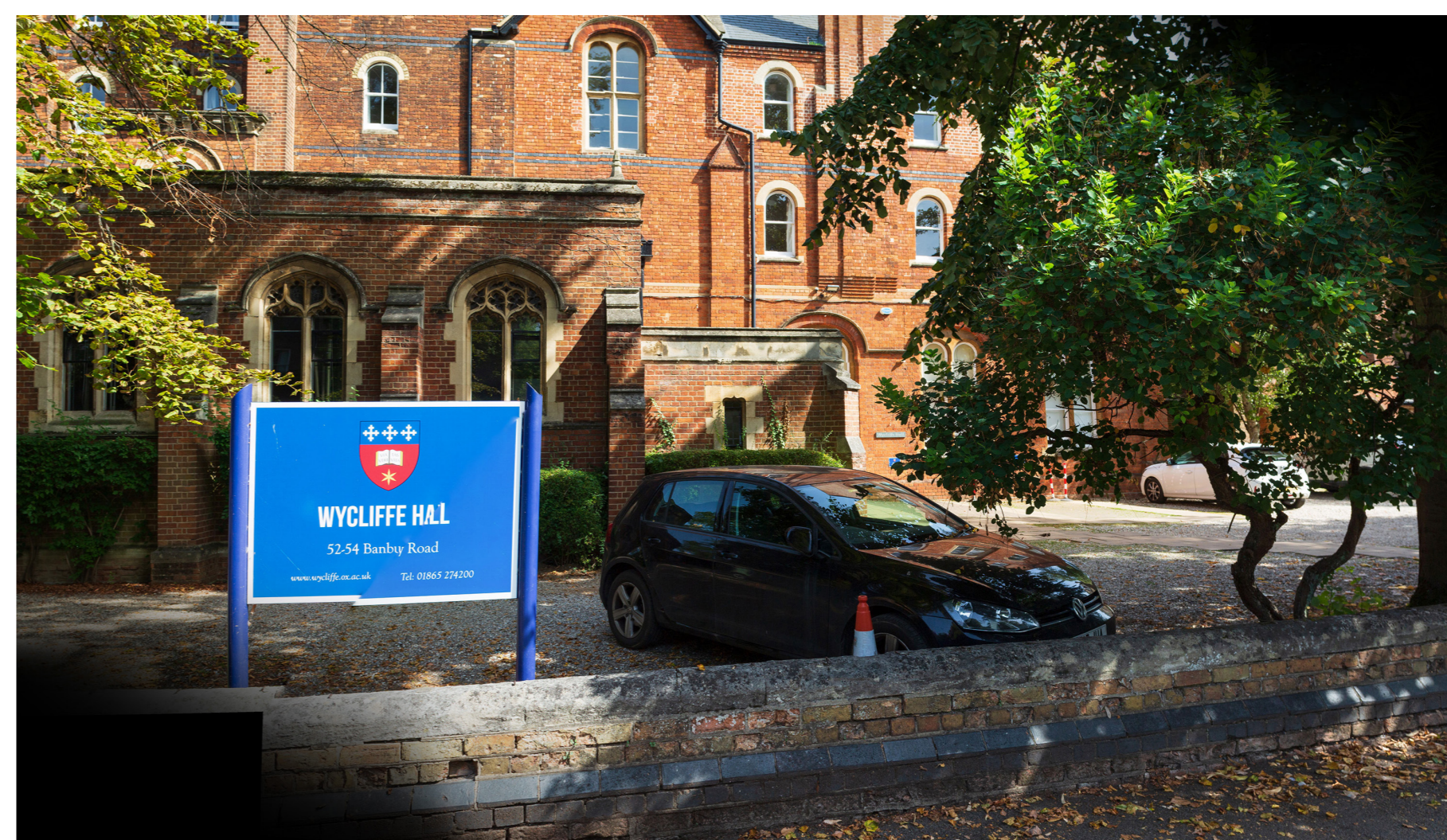
Existing Entrance to Wycliffe Hall
